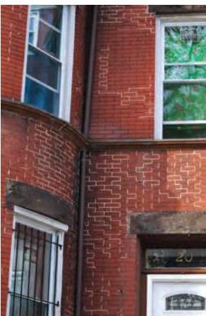
SPOT TUCKPOINTING USING CEMENT
