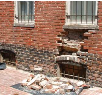
PARTIALLY DEMOLISHED LOAD BEARING BRICK WALLS
